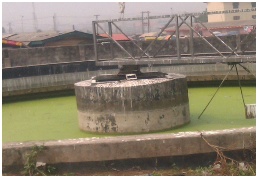
Fig 10. Sewage system at Agege abattoir (Tayo et al., 2016)
